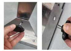
Screw the 4 knobs with short thread (top photo) In the case of larger racks, join the low horizontal bracket and use a fifth short knob (not present in the memmuth 4 rack). Third photo above.
